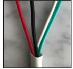
Cut off the excess insulation
